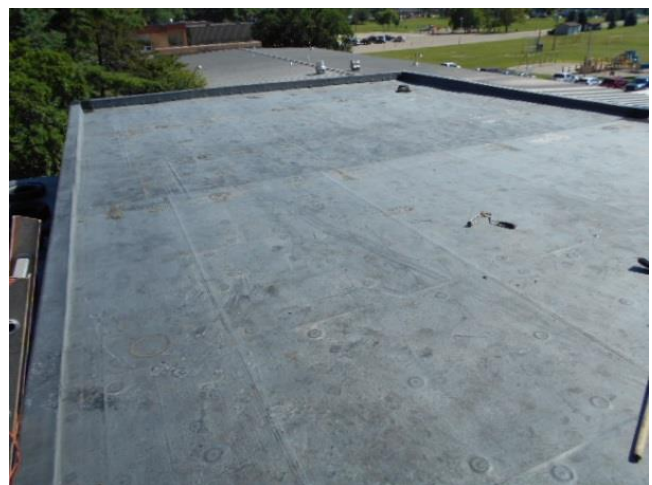
Roof K - Overview
