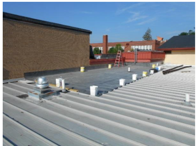
Roof G – In Progress
